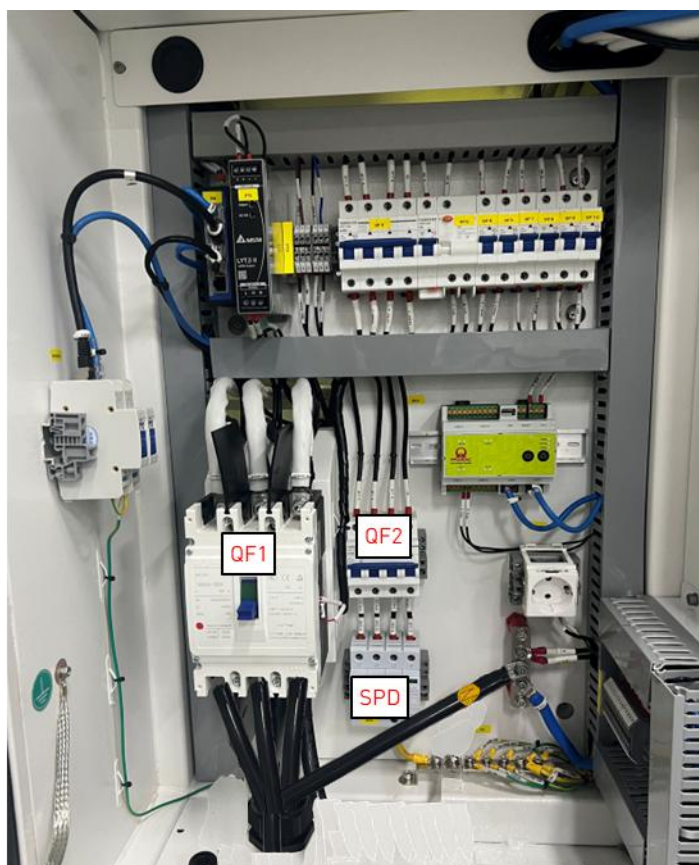
Figure 3-4: Connection AC supply line
